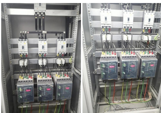
Operating frequency of variable frequency pump at air conditioning side and ground source side
