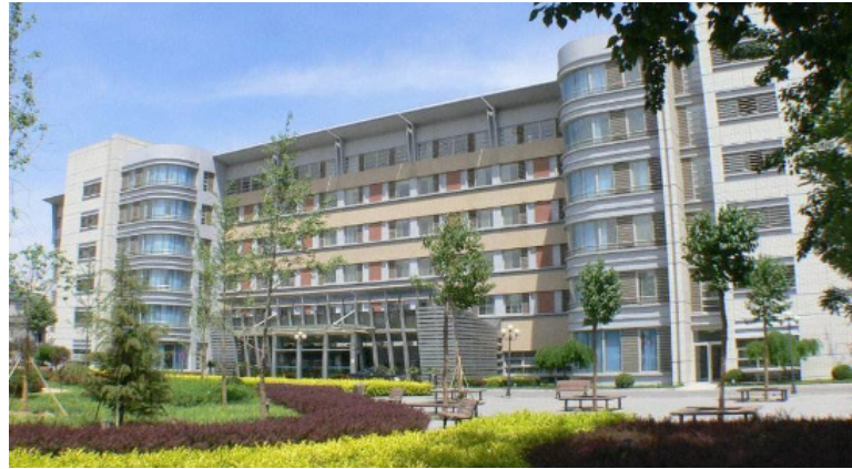
External view of the building
