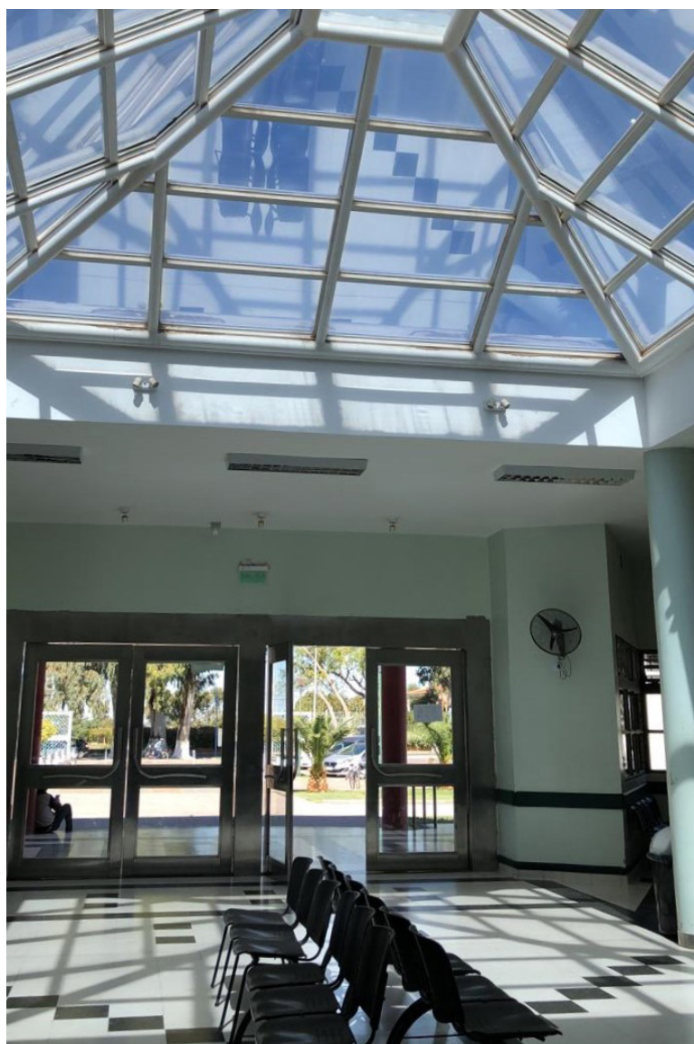
Skylights at Dr. J. Giordano Hospital. San Juan, Argentina
