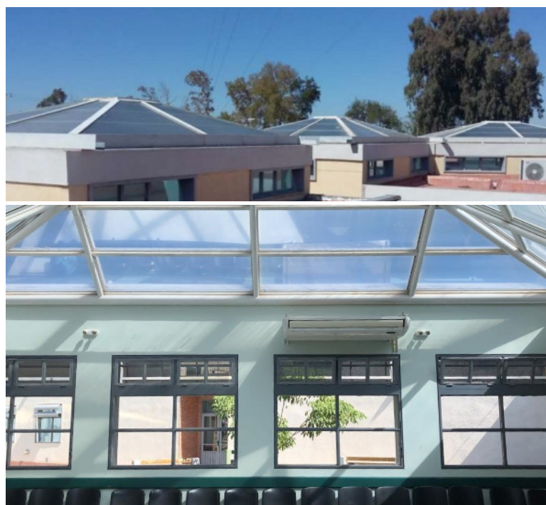
Skylights in Dr. J. Giordano Hospital
