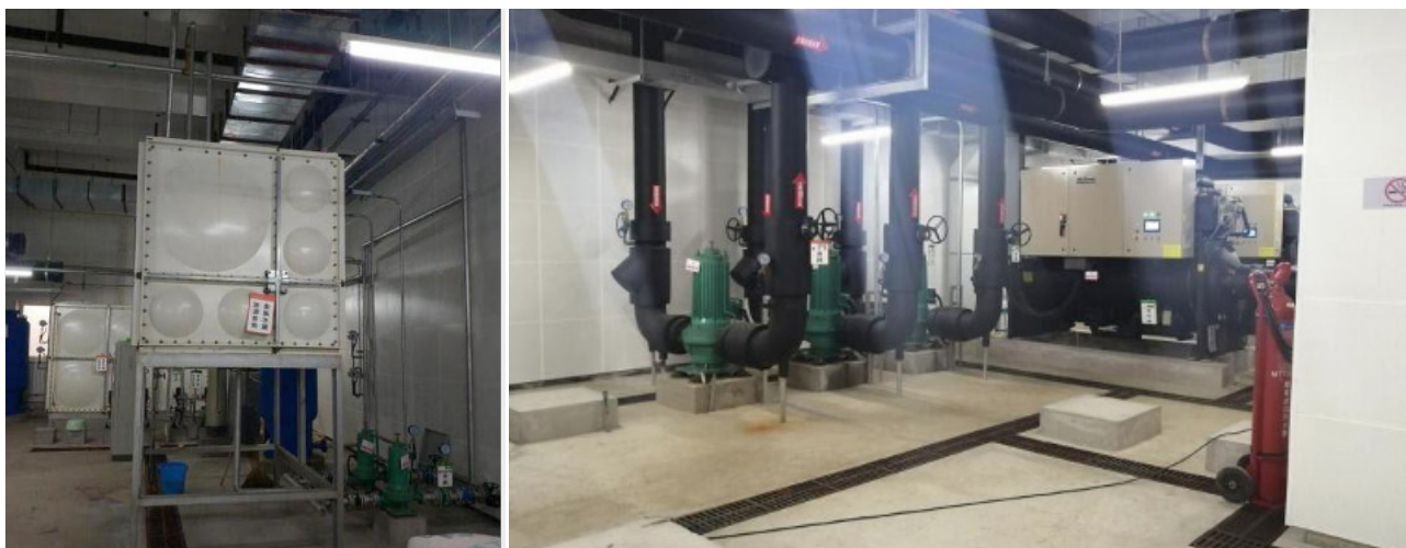
Interior photos of Machine Room
