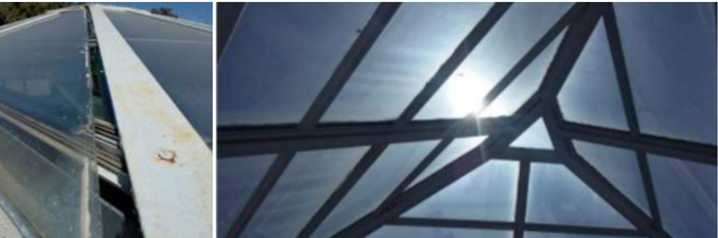
Skylights' air infiltration and incoming light through the structure
