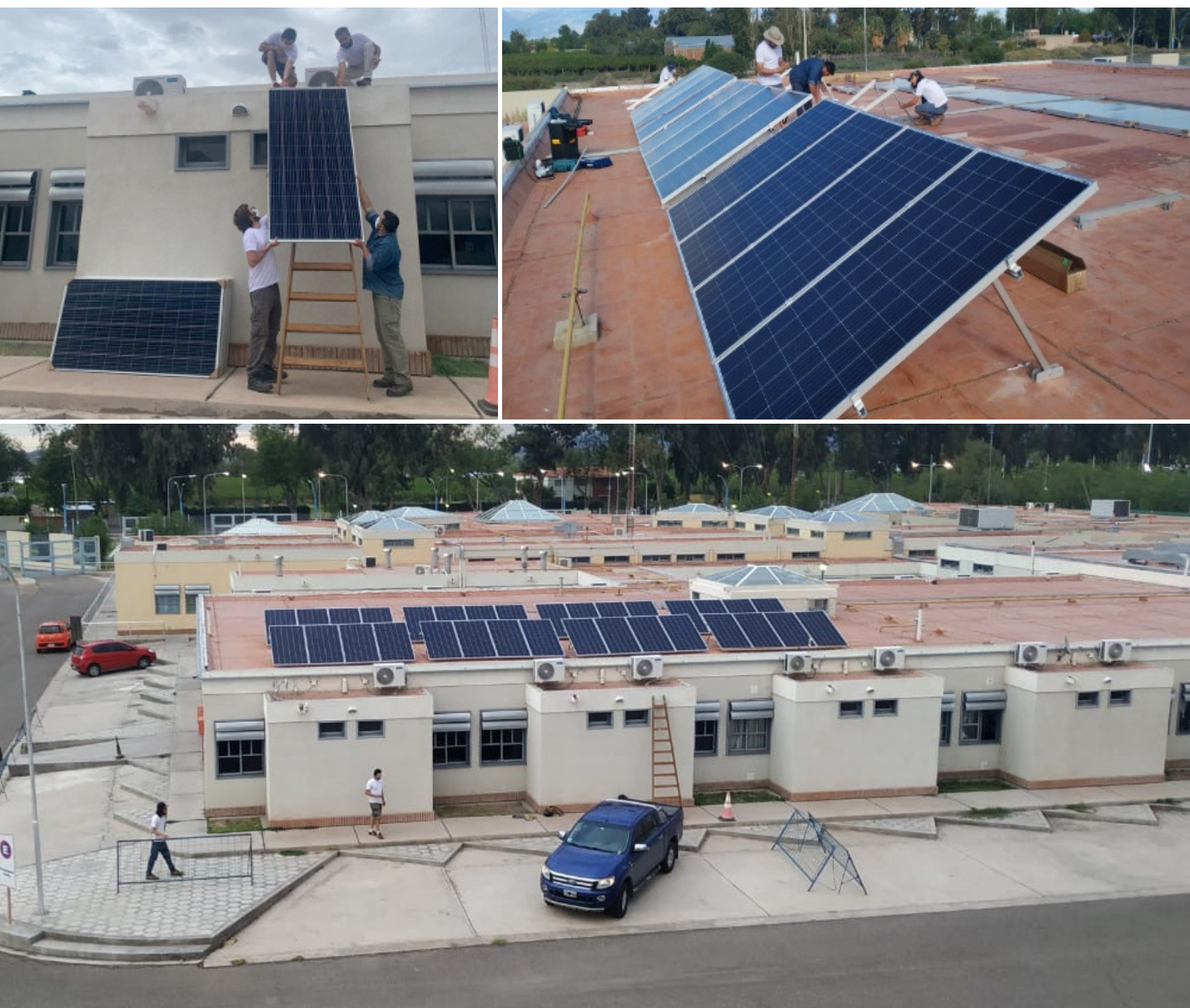
Installation process of photovoltaic energy equipment in Dr. J. Giordano Hospital
