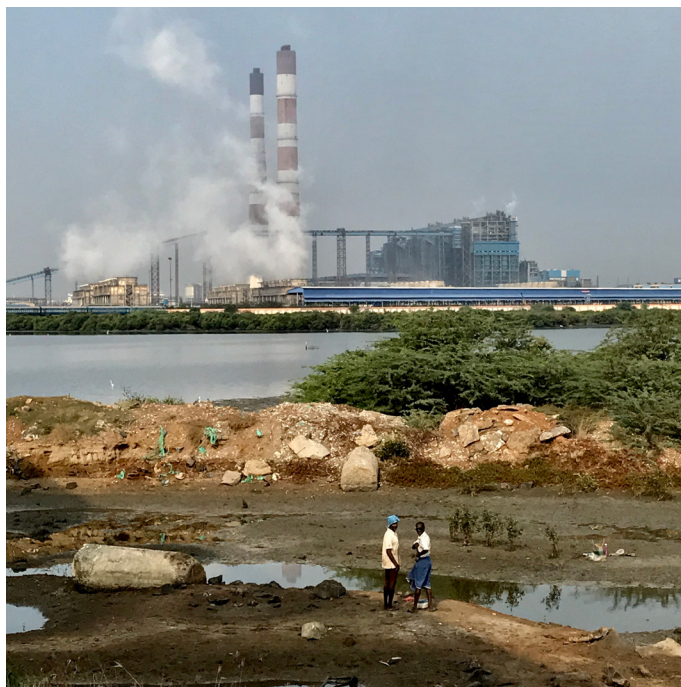
View of the Ennore Thermal Power Station. Photo: Health Care Without Harm
