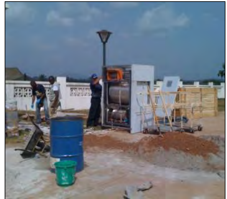
Installation completed in 1 day
