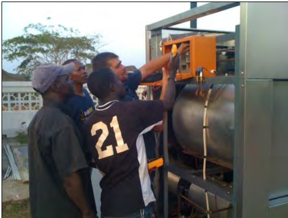
Training maintenance and repair technicians during the installation
