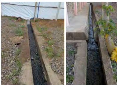
Figure 11. Open wastewater channels in the green zone (left) and red zone (right) of two ETUs
