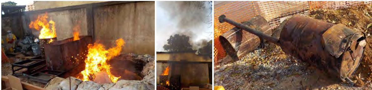
Figure 14. Burn barrels and burn pit in the red zone of an ETU; the yellow colored building behind the wall a few meters from the burn pit (center photo) is the ward for confirmed Ebola patients; photo on the right shows two previous burn barrels used
