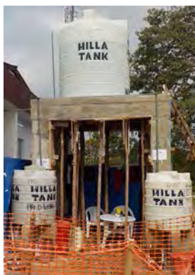
Figure 28. Large plastic containers of hypochlorite solutions under the sun
