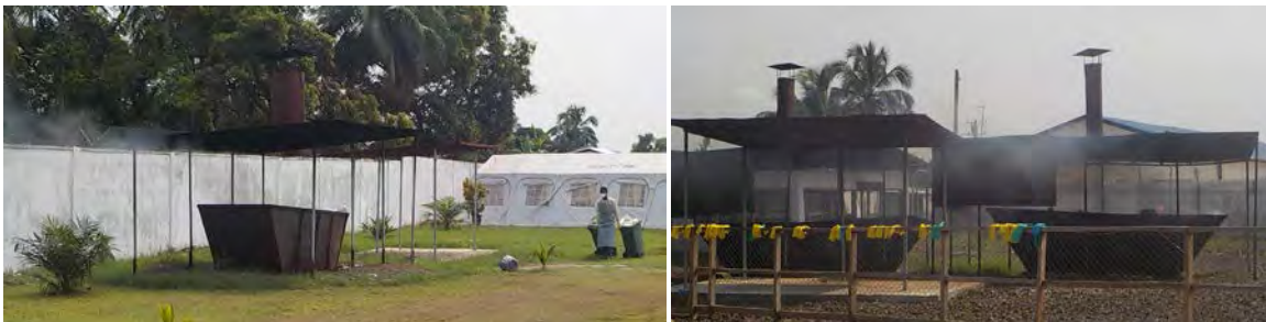
Figure 15. Large burn skip on the green zone (left) and red zone (right) of an ETU; the two red zone burn skips (right photo) were about 15 meters from the Ebola patient wards
