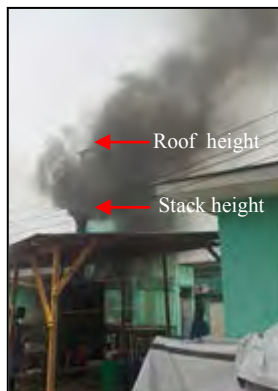
Figure 20. Chimney of an incinerator several meters below the top of a nearby building (partially covered by smoke)
