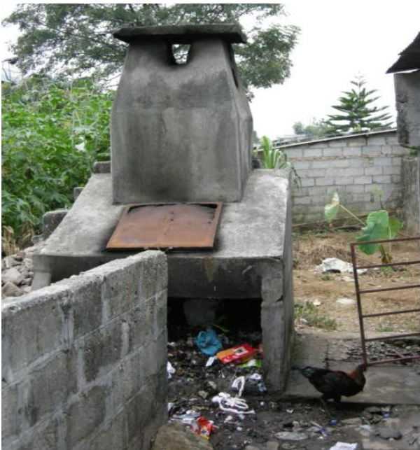
Small scale hospital incinerator in Nepal. A chicken hunts for food nearby (Nakarmi/HECAF).
